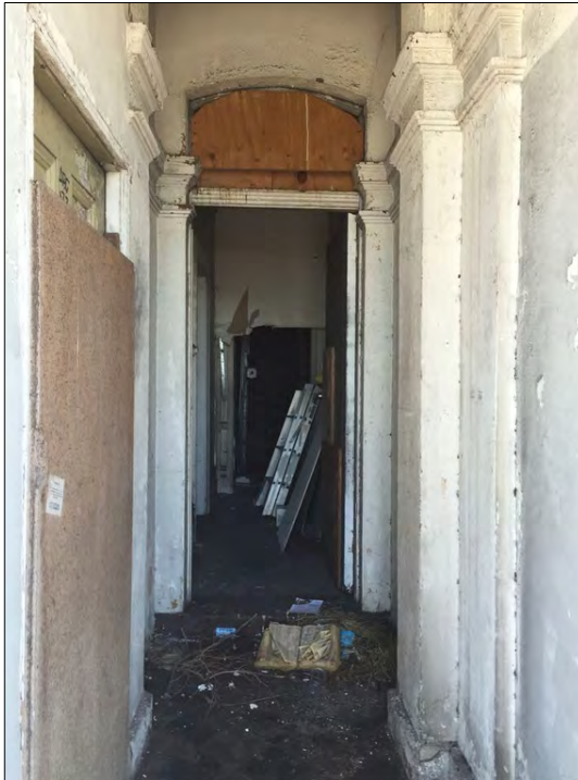
Figure 35: Ground floor hallway.
