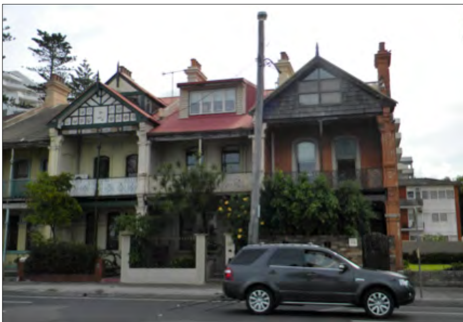
Figure 15: Street front elevation of (from left to right) Nos. 67, 66, 65 and 64 The Grand Parade.
