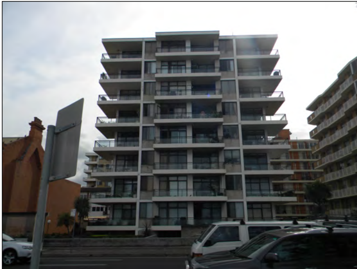
Figure 64: No. 58-63 The Grand Parade, an eight storey 1970s residential tower.
