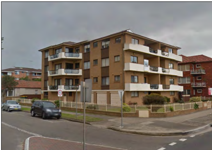
Figure 66: No. 51-54 The Grand Parade, a late twentieth century residential flat building on the corner of Gordon Street and The Grand Parade. Google Maps.
