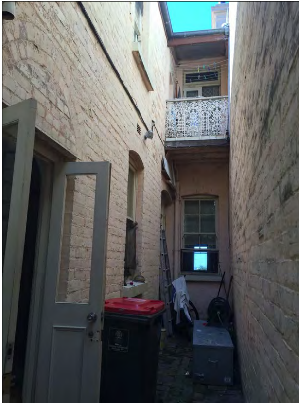
Figure 21: Rear of No. 67 The Grand Parade. Architecture and Building Works.
