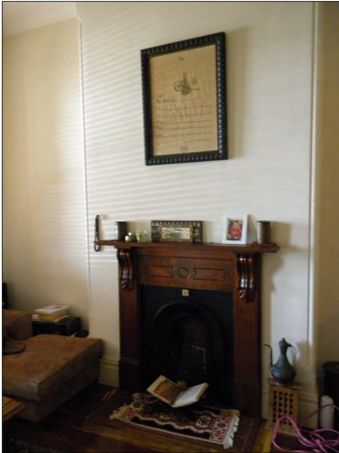
Figure 37: Ground floor, front room, showing the cast iron register grate and timber chimneypiece.
