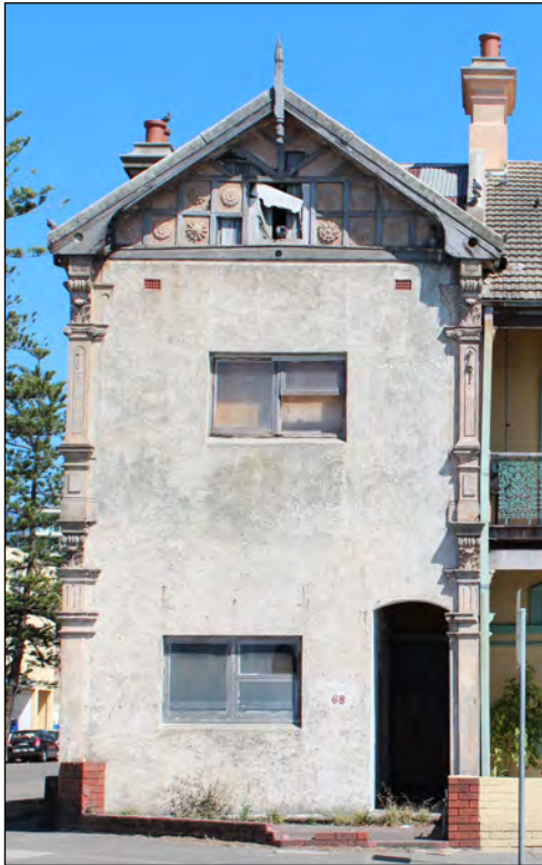
Figure 16: No. 68 The Grand Parade from the street. Architecture and Building Works. Modified by Weir Phillips.
