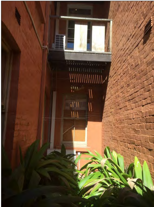
Figure 31: Rear of the principal building form. Architecture and Building Works.
