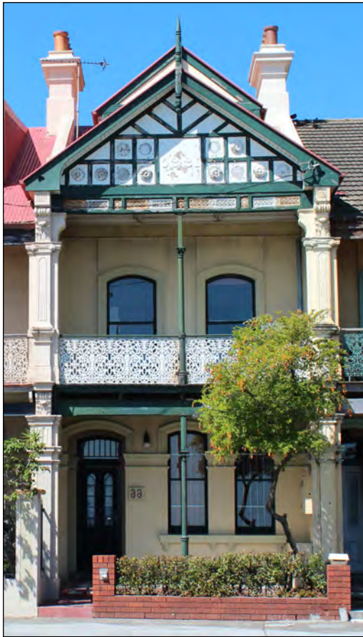
Figure 23: Street view of No. 66 The Grand Parade. Architecture and Building Works. Modified by Weir Phillips.
