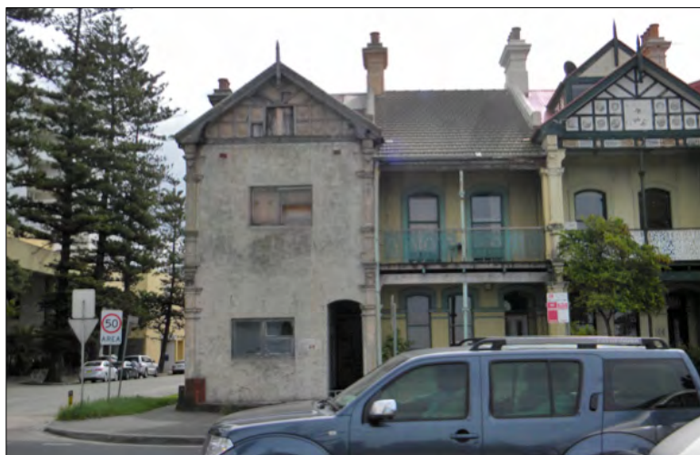
Figure 13: Street front elevation of (from left to right) Nos. 68, 67 and 66 The Grand Parade.
