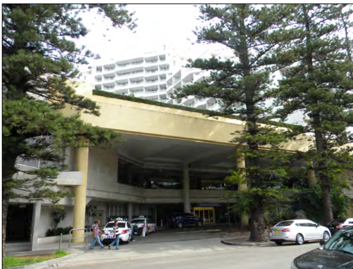
Figure 68: The vehicle entrance and parking bay at the rear of the Novotel Hotel facing onto Princess Street.
