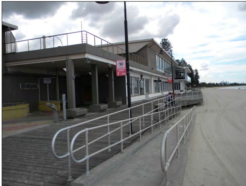
Figure 75: View of the east elevation of the Brighton Baths.
