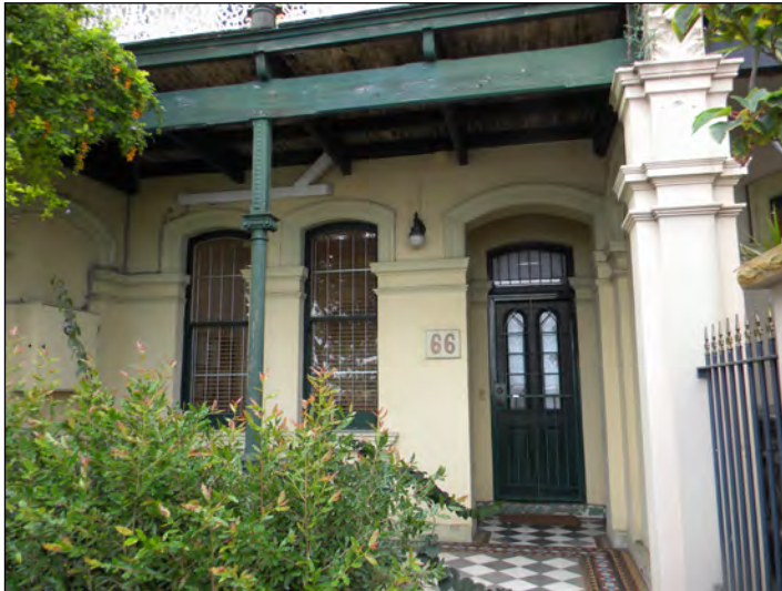
Figure 24: View of the ground floor verandah and elevation of No. 66 The Grand Parade.
