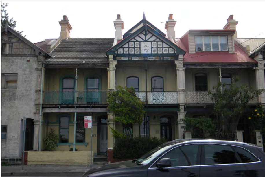
Figure 14: Street front elevation of (from left to right) Nos. 68, 67, 66 and 65 The Grand Parade.
