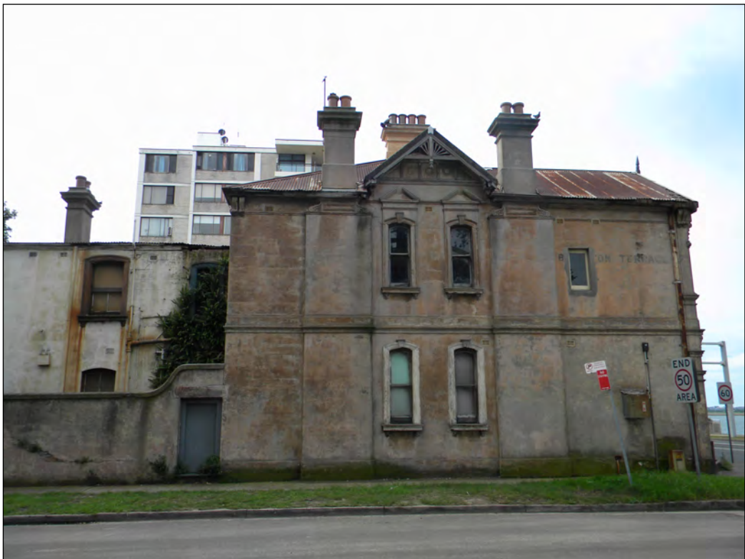
Figure 17: South elevation of No. 68 The Grand Parade viewed from across Princess Street. This is the only wing along the row still retaining its original chimney.
