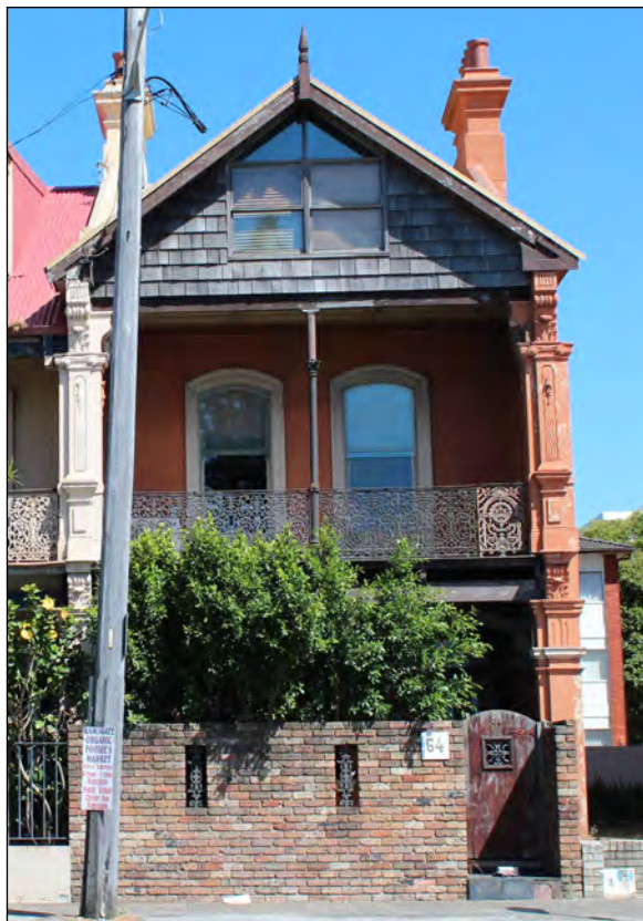
Figure 28: Street view of No. 64 The Grand Parade. Architecture and Building Works. Modified by Weir Phillips.
