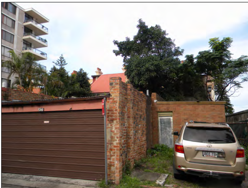
Figure 19: Rear yard showing the uncovered car space.
